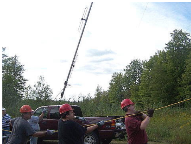
The ground crew starts pulling up the new antenna
