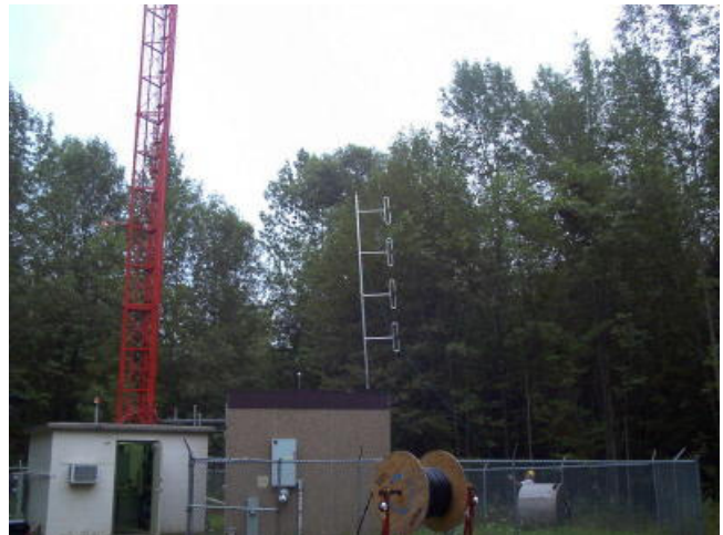
The new repeater antenna on the way up the tower
