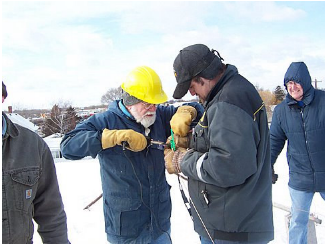
Ken, N0AWM solders the feedpoint of the new 80-meter loop at the DAR. W9DWG assists, K8IR tries to stay warm
